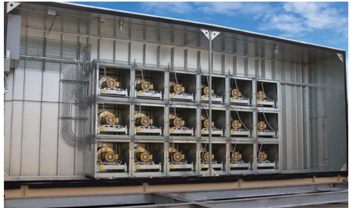
**Direct-Drive Plenum** fan arrays allow up to 100 percent redundancy for greater systems reliability and up to 10 percent increased efficiency.
